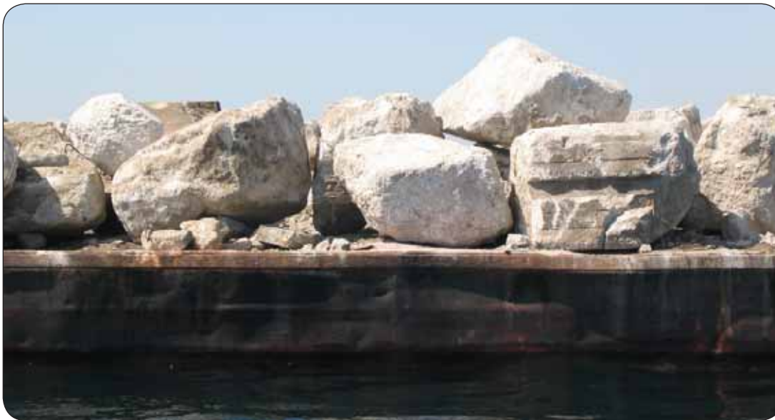
A barge load of demolition concrete. One barge load can contain 500 to over 5,000 tons of material.
